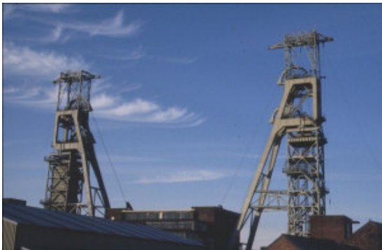
Headgear at a disused UK coal mine Photo Copyright: BGS©NERC
